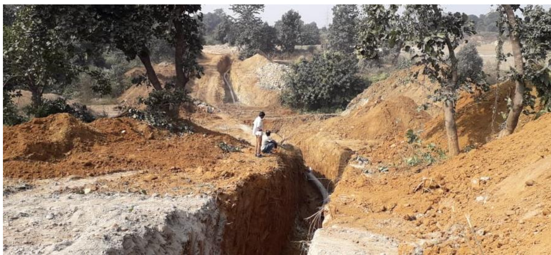
Pipeline laid for a Cross-Country Project
