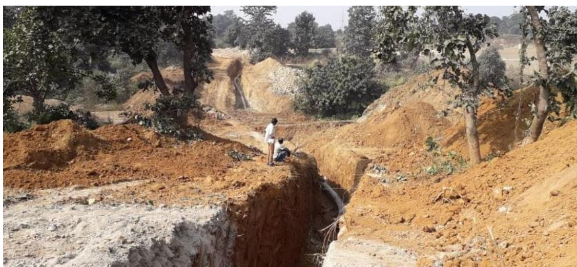
Pipeline laid for a Cross-Country Project
