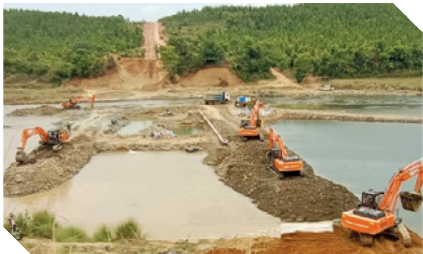
↑ Open Cut Method- Dhobi Durgapur pipeline project
