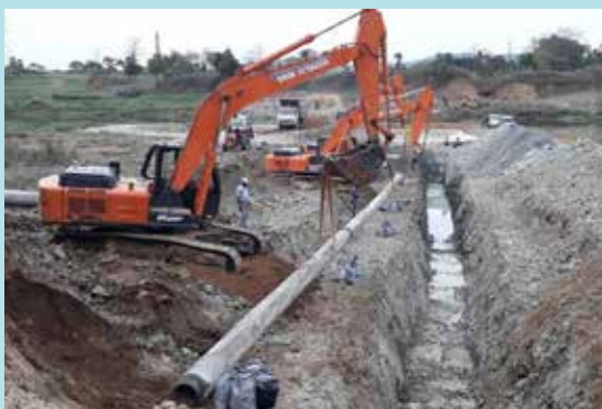
Cross-Country Pipeline Projects (CCP)
